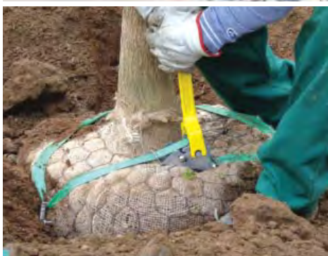
Tree Anchoring Systems: Deadman Systems - Plati-Mat® & Strap
